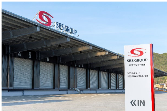
Exterior view of Logistics Center Kirishima
