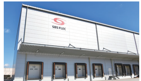
Ami Low Temperature Logistics Center
