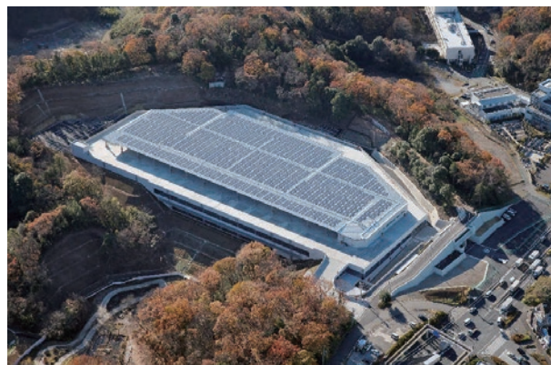
Nagatsuta Logistics Center (commencing operations in spring 2015)
