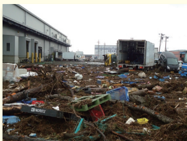
Iwanuma Logistics Center just after the disaster
