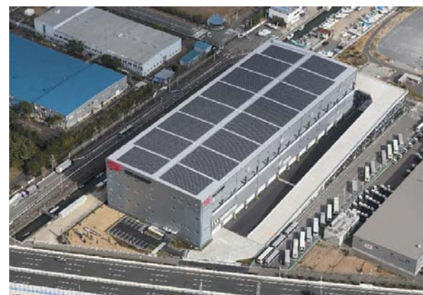
Solar power generation equipment installed on the roof of the Sinsugita Logistics Center of SBS Logicom (completed February, 2016)
