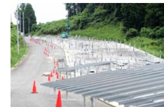
Shibayama No. 2 under construction
