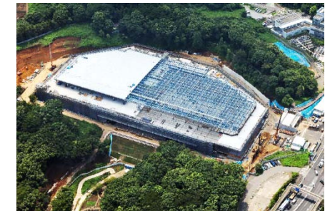
Construction under way at Nagatsuta Logistics Center in Yokohama
