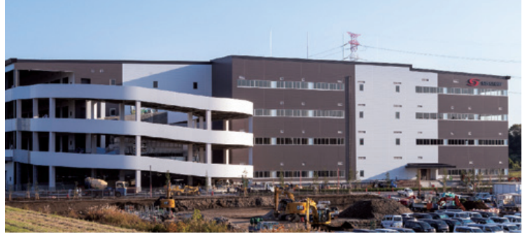
Building A of Noda Seto Logistics Center
