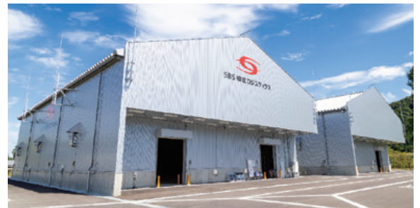
Kashiwazaki Warehouse, Kashiwazaki Logistics Center
