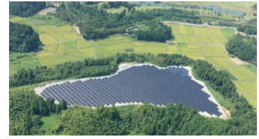
Shibayama Solar Power Plant
